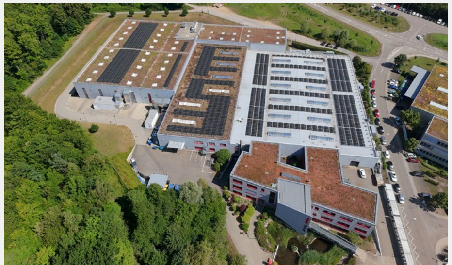
The PV system covers almost 3,200 square metres of MAPAL's roof in Pforzheim. Renewable energy now covers 12 percent of the entire power requirement of the location.
